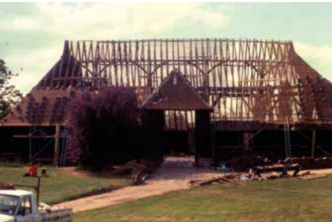
Photograph 37: The biggest medieval buildings that could be built from ordinary trees were the great barns. This one was built c. 1200 CE from some 450 mostly small oak-trees. It was a storehouse for the agri-business of the Knights Templars, military monks (Cressing Temple, Essex, England, 1989).
