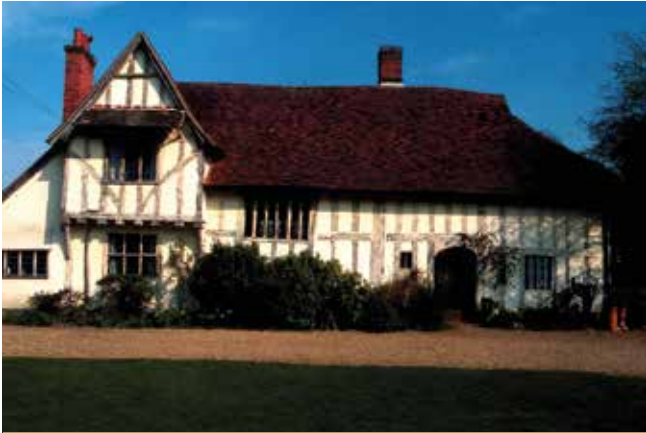
Photograph 36: An ordinary timber-framed house of c. 1400 CE. The timber frame is made partly of cheaper species than oak, and of recycled timbers. The spaces between the timbers are filled with coppice poles covered with clay (Flatford, Suffolk, England).
