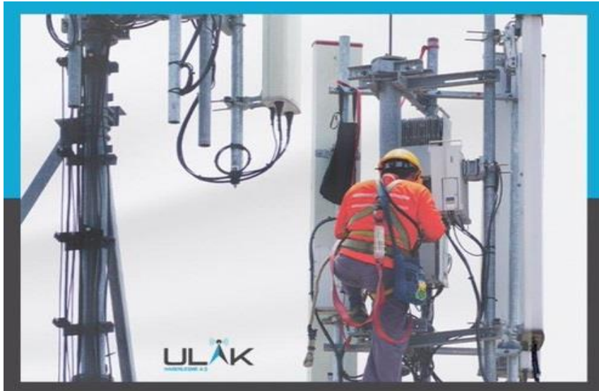
Figure 3. Installation of Ulak Base Station.
